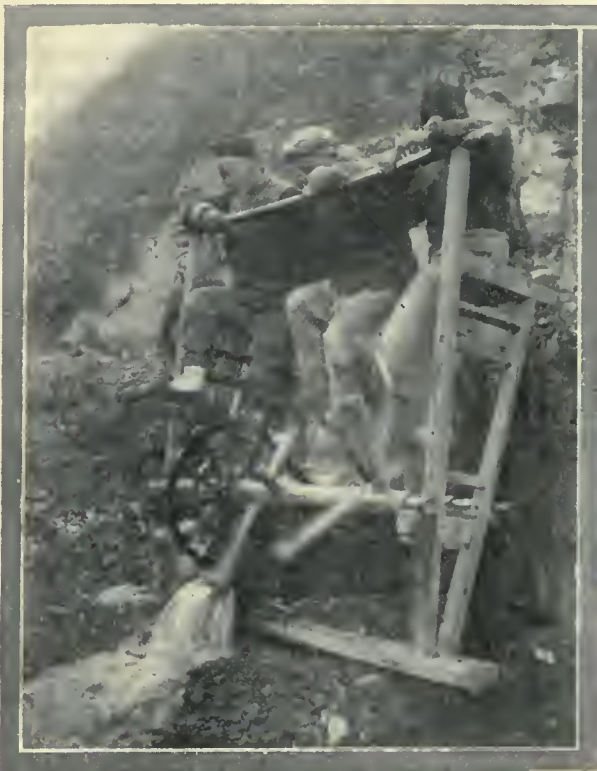
PUMPING OUT A PROSPECT HOLE.
